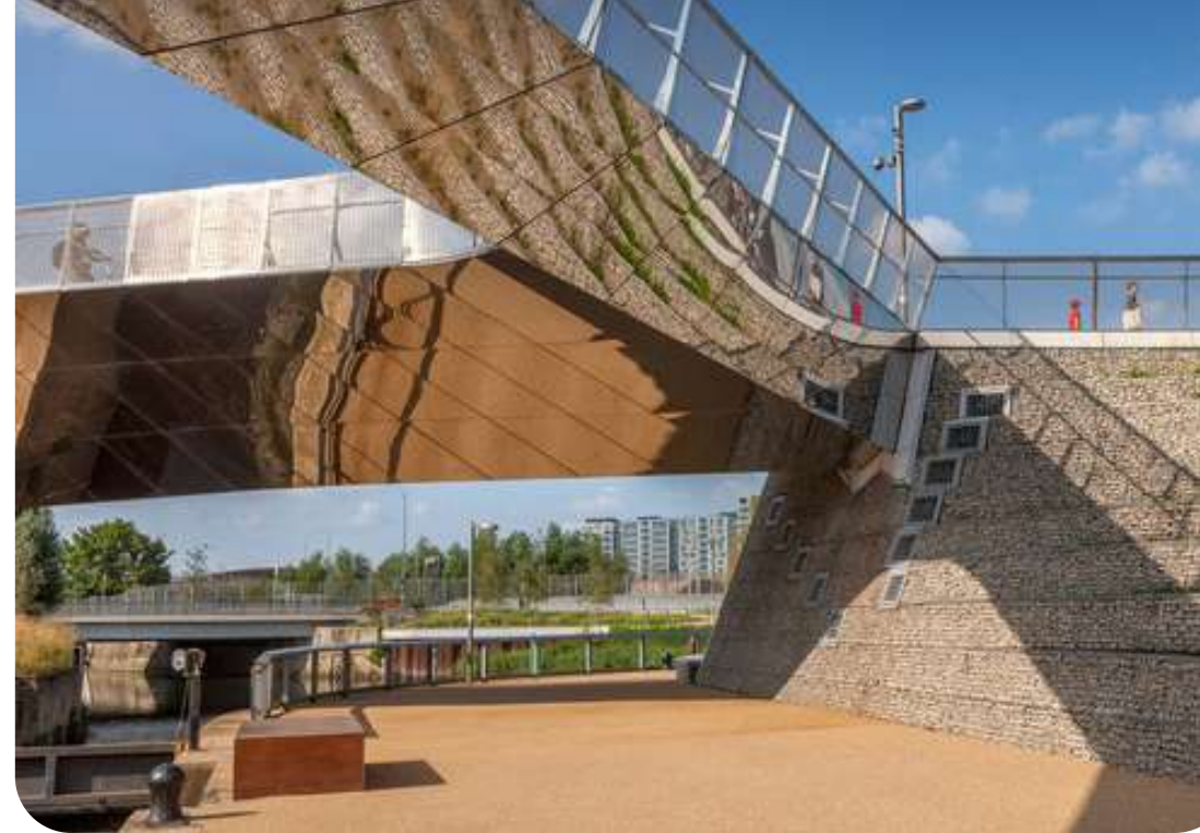
Contemporary canal bridge, Queen Elizabeth Olympic Park, London
