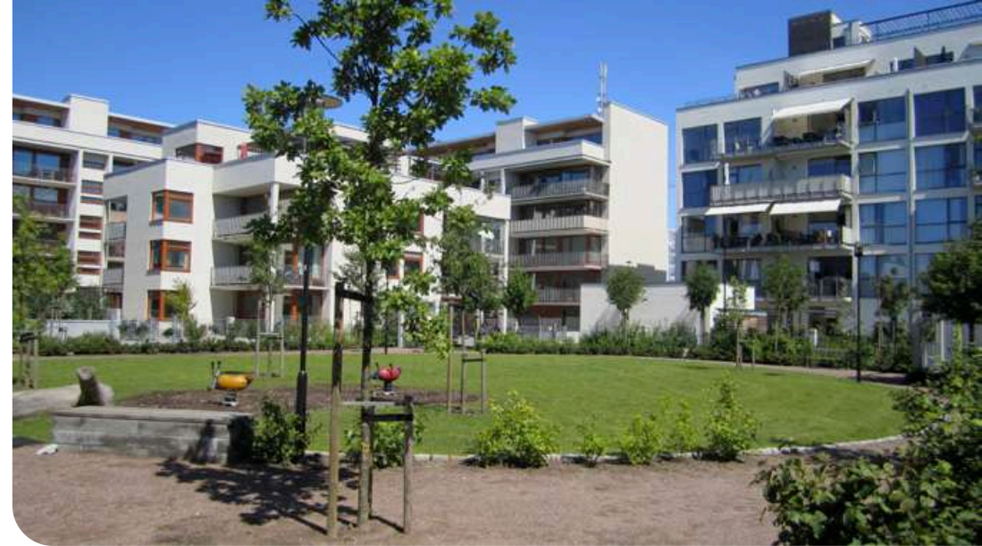
Communal open space which is large enough for children to run around and include a small play area, trees, planting and places to sit, Malmo, Sweden. © La Citta Vita
