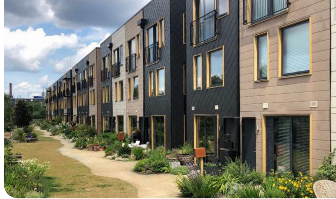
The Climate Innovation District in Leeds (above) was designed as a powerful response to climate change through embedding passive and climate responsive design techniques, harnessing the sites natural resources and delivering highly energy efficient and resilient homes.
