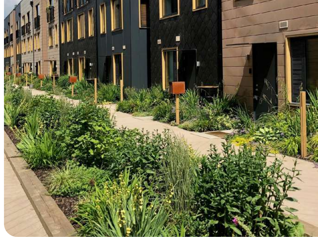
Raingardens incorporated within streets and hard impermeable surfacing kept to a minimum, Leeds Climate Innovation District.
