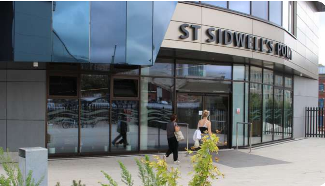
St Sidwell's Point Leisure Centre, Exeter. The first leisure centre in the UK built to Passivhaus standards.
